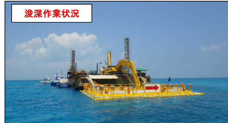
汚濁防止枠 (14m × 14m)
